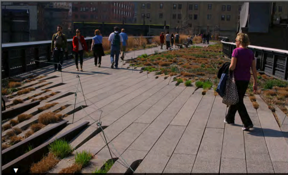
Diagonal Concrete planks taper into planted areas; the designers' goal was to blur the edges between pavement and plantings.
