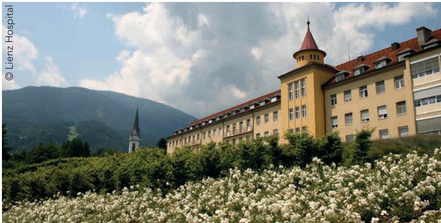
Lienz Hospital in East Tyrol, Austria.
